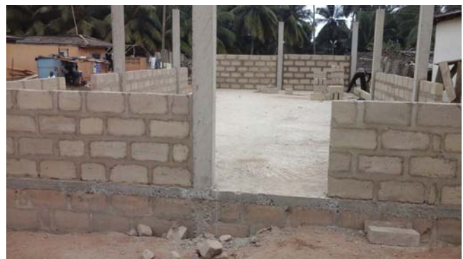
Figure 2. Construction of the community centre underway in Ghana (Photo: Andrews Agyekumhene)
